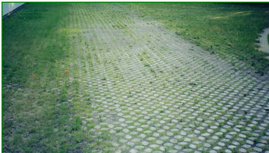
Figure 1 Porous Pavement – UAA Arts Building
